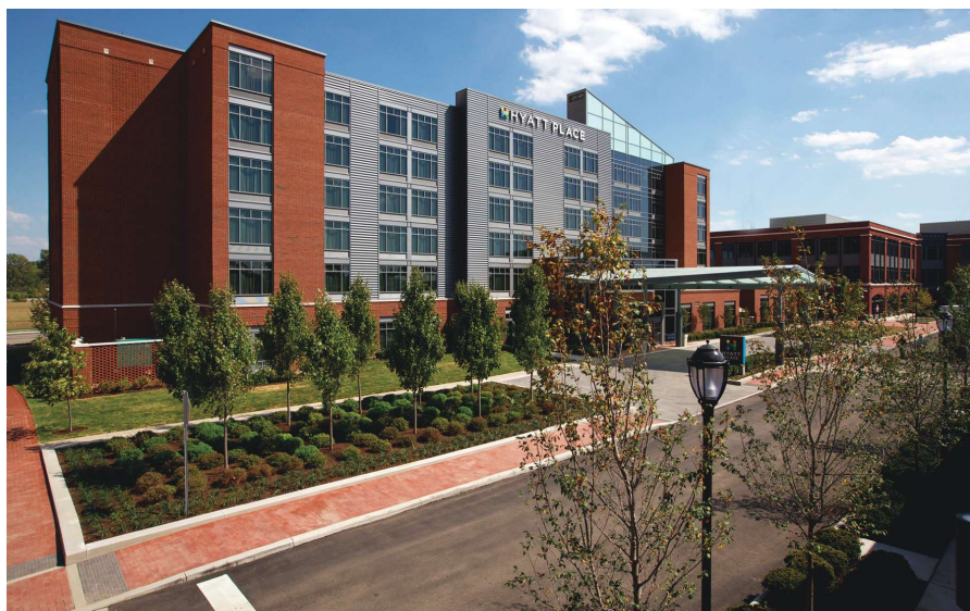
A 126-room Hyatt Place is part of Grandview Yard.
