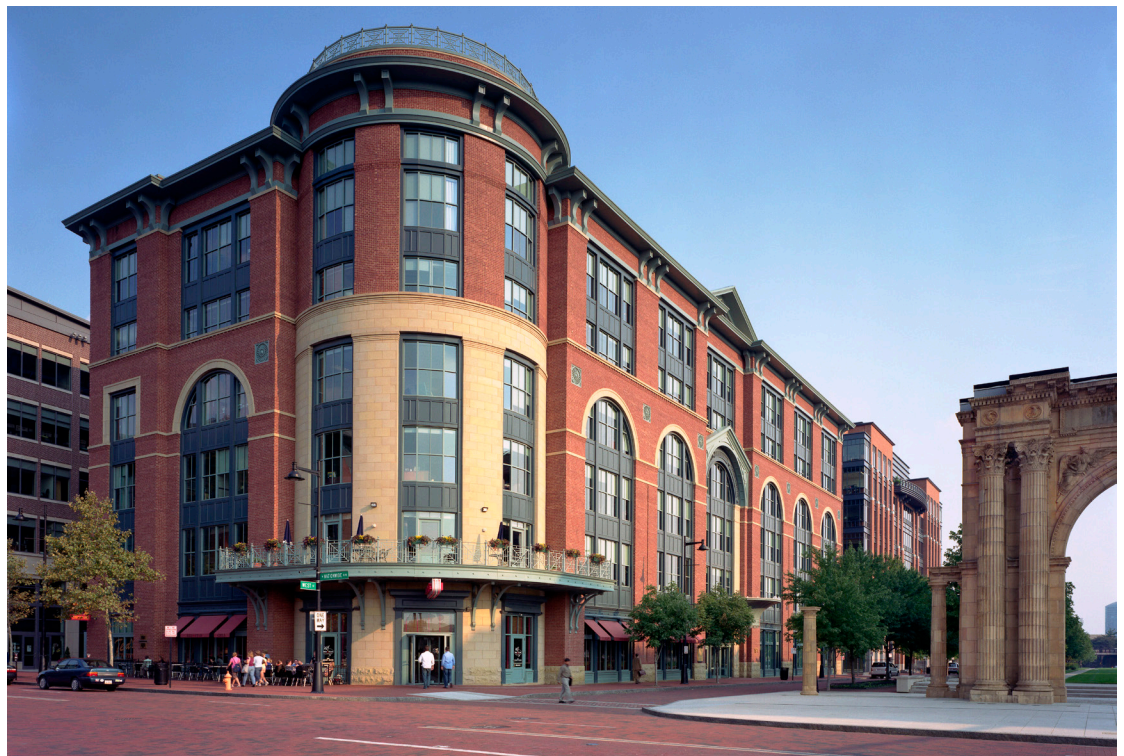
The Arena District in Columbus features more than 1.5 million square feet of commercial space including the six-story, 134,000-square-foot 191 Nationwide Boulevard building. The ground floor offers 21,000 square feet of the Arena District's most visible retail and restaurant space.
