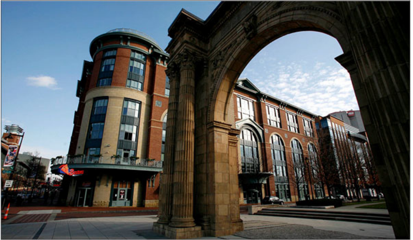
The Columbus Arch was part of an old railroad station near the new Arena District, a riverfront development.
