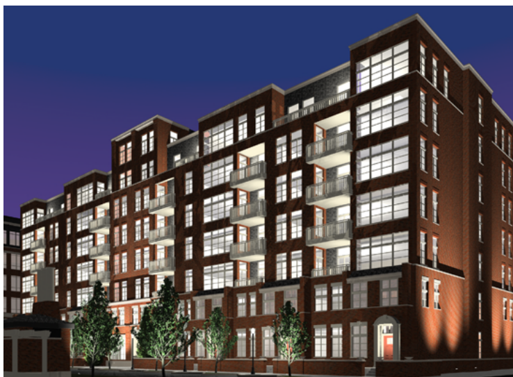
Two eight-story buildings called Arena District condominiums, pictured in a rendering, are planned by Nationwide Realty Investors. The asking price will start at $249,000.
