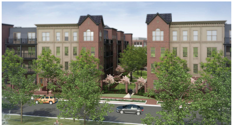
The final 40 acres of development in the westernmost reaches of the Arena District will be devoted largely to apartments and condominiums.
