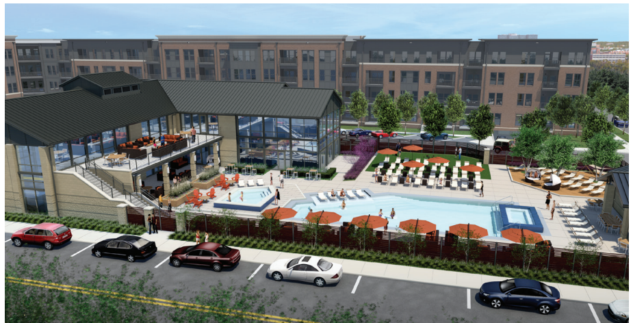
The Yard Club residential amenity building is underway and will be open to residents later this summer.
