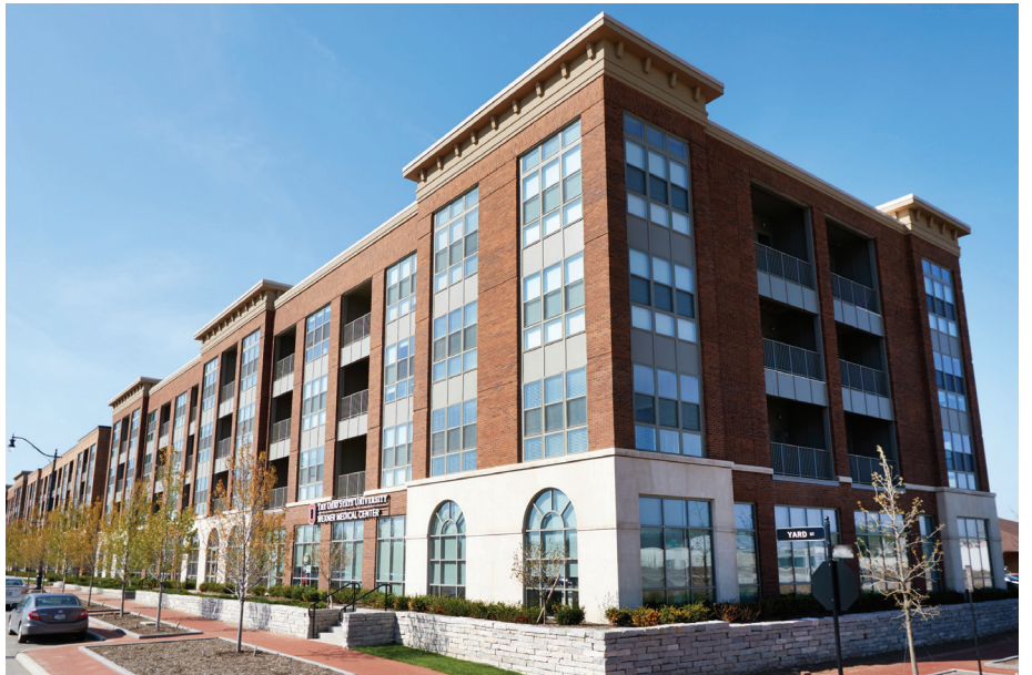
Grandview Yard continues to expand in Grandview Heights, a first ring suburb of Columbus, Ohio.
