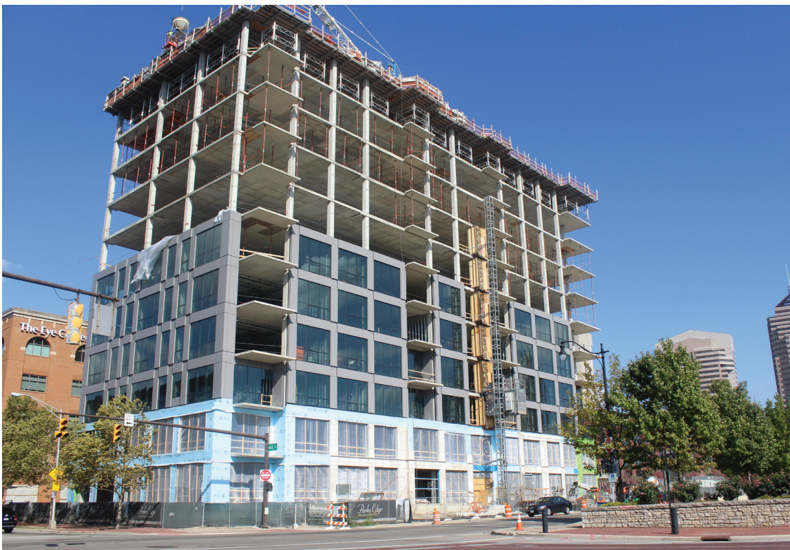
The building as it looked in October.
